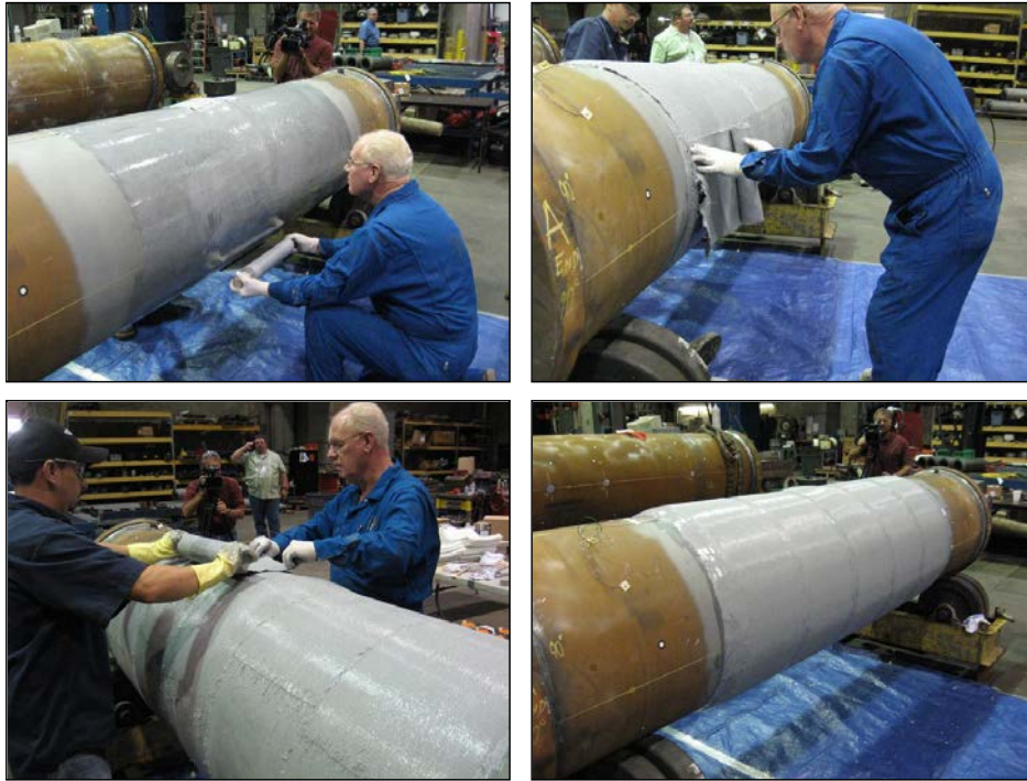
Figure 8 – Photographs showing installation of composite materials on wrinkle bend samples
