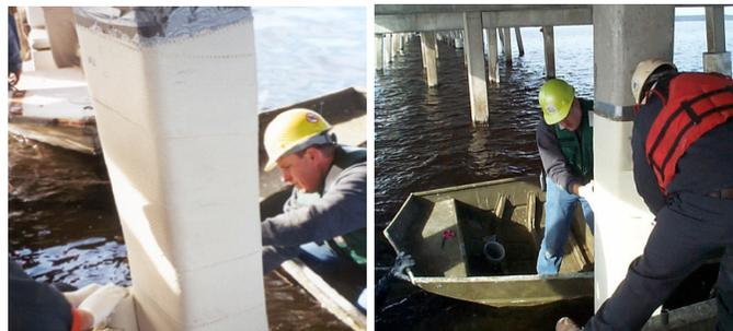
Figure 6. Aquawrap® installation
