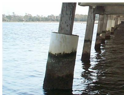
Figure 4. Concrete Encapsulation
