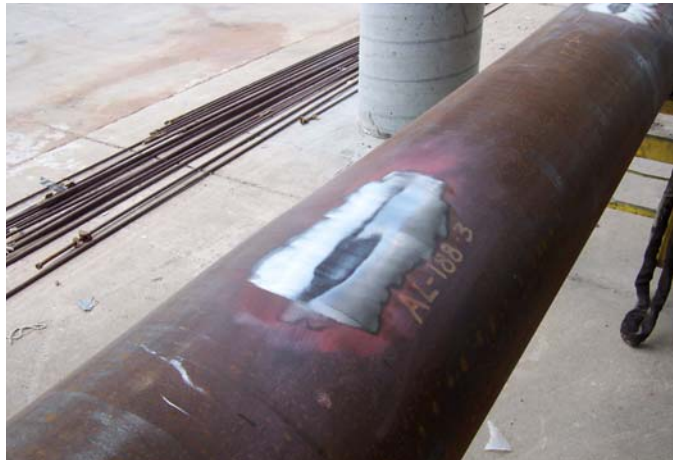
Figure 3 – Gouge removal by grinding
