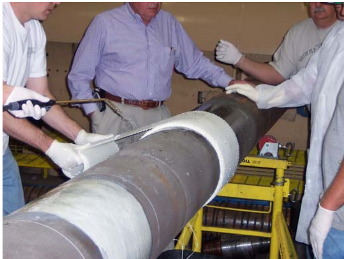
Figure 4 – Installing composite material on pipe
