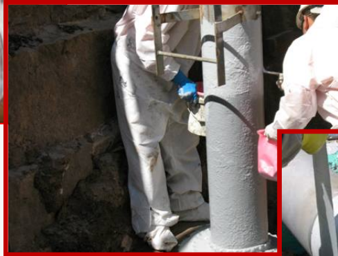
Apply to Pipe Surface
