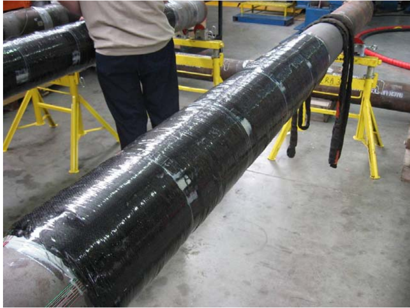
Figure 10 – Final view of cured repair prior to testing
