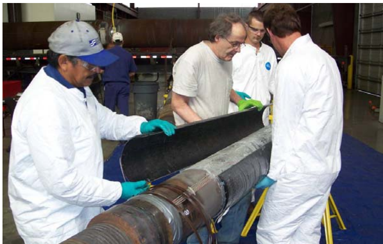
Figure 9 – Installation of the carbon half shells
