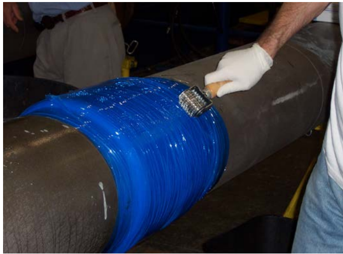
Figure 5 - Perforating plastic wrap to permit off-gassing during cure
