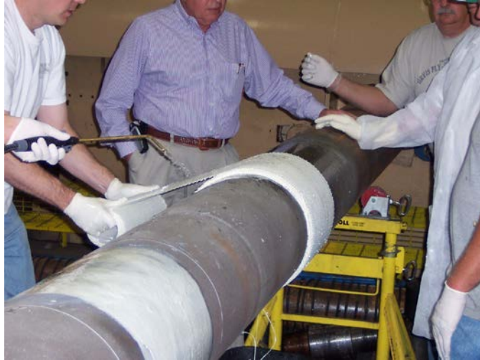
Figure 4 – Installing composite material on pipe
