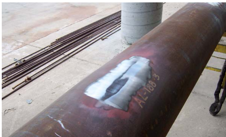
Figure 3 - Gouge removal by grinding
