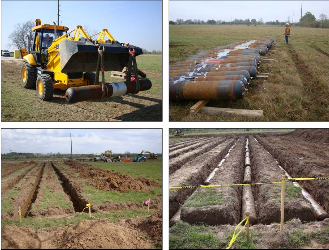
Figure 5: Photographs from pipe burial for the long-term study
